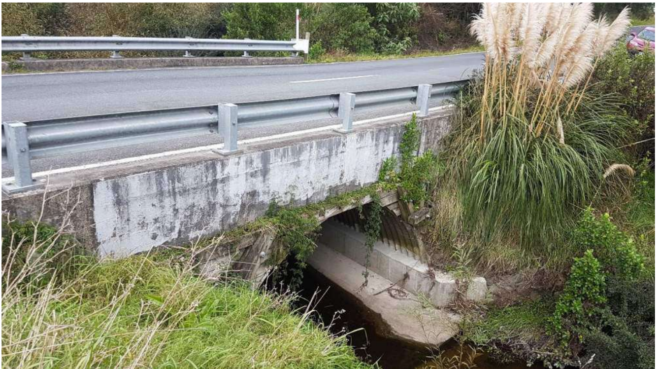
Photo 7: Small Road culvert downstream of the Structure Plan Area
