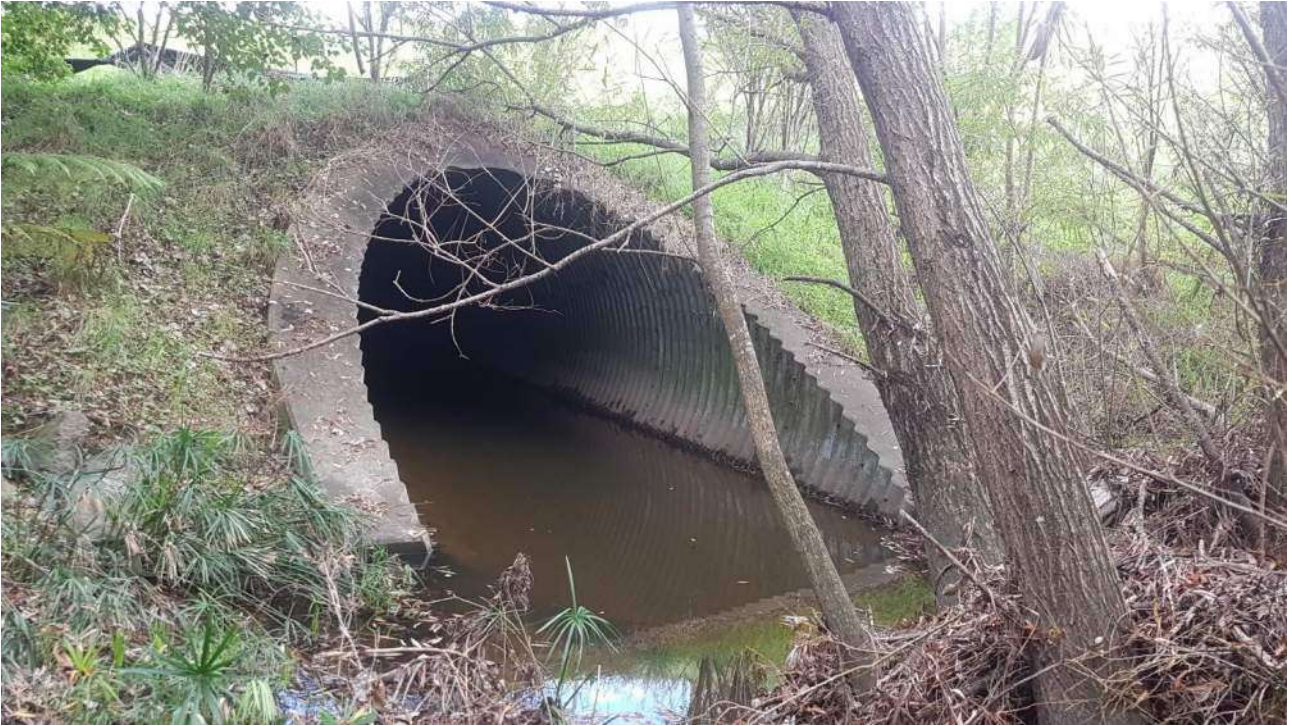
Photo 3: SH1 Culvert (downstream end) at Silverdale Interchange
